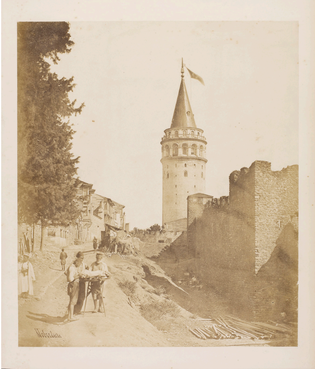
Figure 4. The walls of Galata before the demolition.
